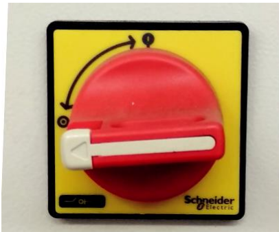
Figure 40 Main electric switch
