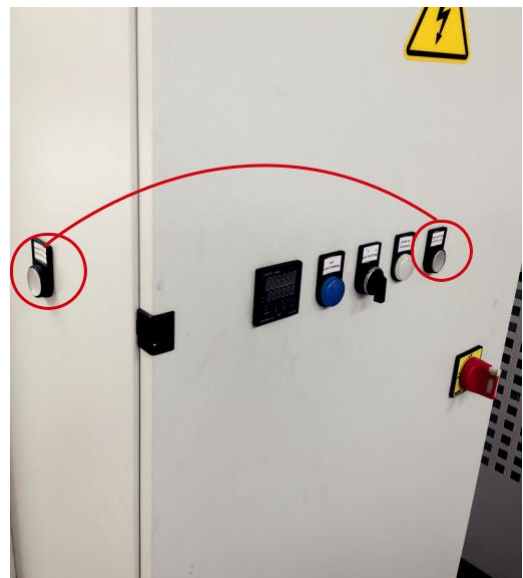
Figure 39 Photocell Reset Buttons
